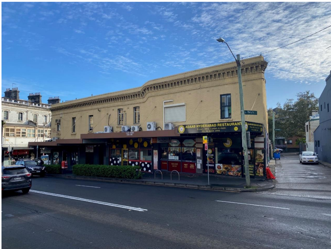
Figure 2: Site viewed from the opposite side of Cleveland Street looking north
