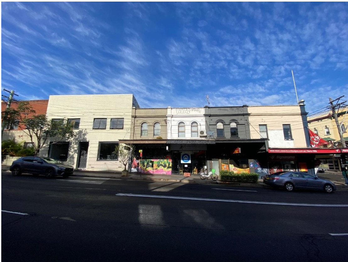
Figure 14: Neighbouring development on the opposite side of Cleveland Street, looking south
